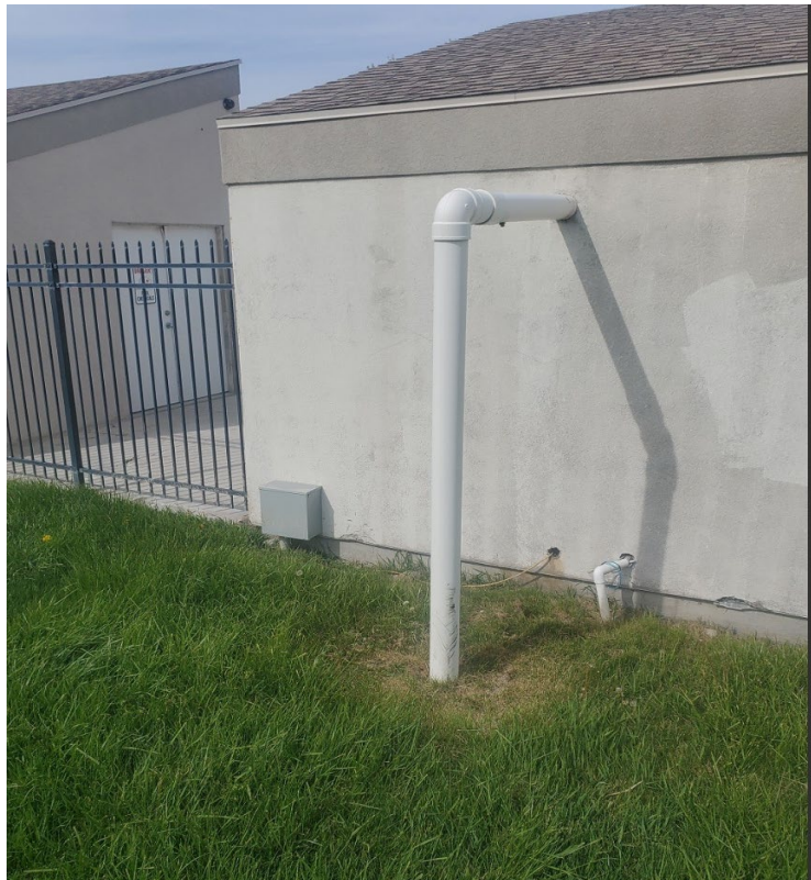
Backflush Effluent Pipe from Mechanical Room
